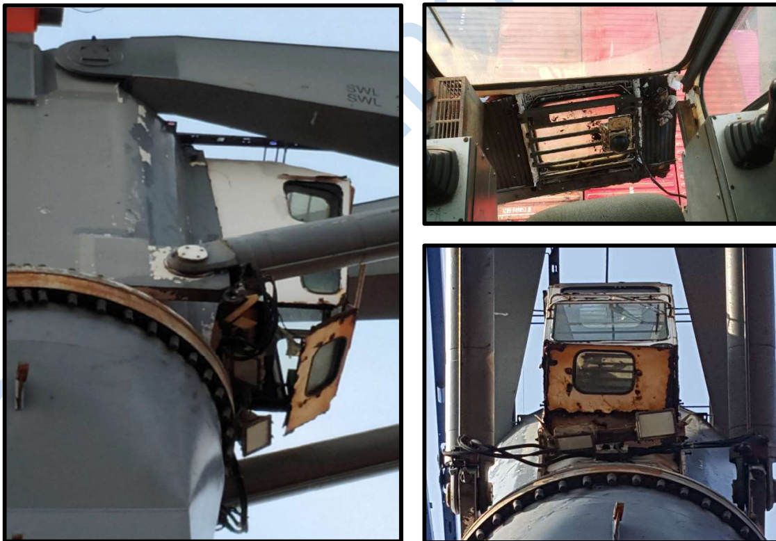
Picture 2: Photograph of the base plate of the crane cabin taken after the accident
